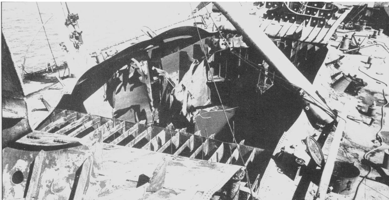
*Figure 1: Example of tanker explosion damage*
